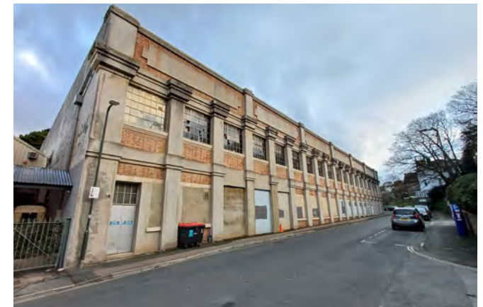
The east elevation of the former interwar coach depot, between Torwood Street and Torwood Gardens Road.
