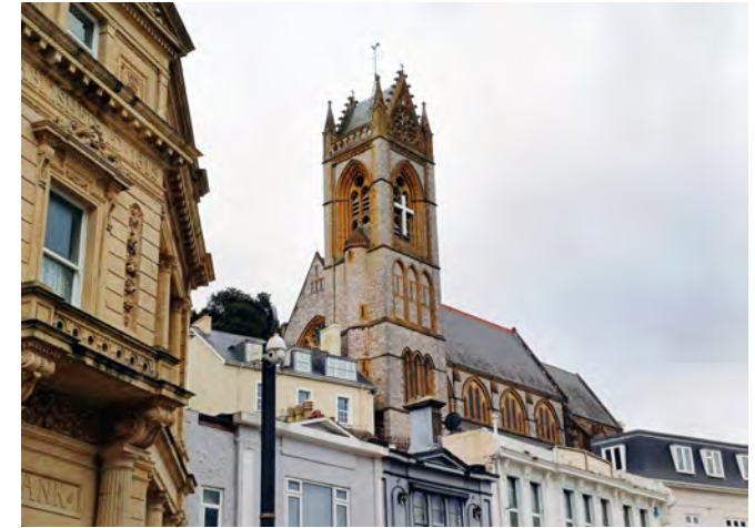
Church of St John the Evangelist, built between 1861-73 with a west tower of 1884-85, viewed from Fleet Street.
