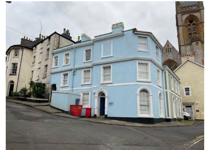
Georgian houses on the corner of Montpellier Road and Braddons Hill Road West.
