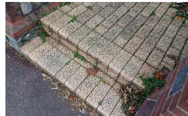
Hard-fired, cream coloured clay pavers surviving to the front steps of a property on Babbacombe Road. The pavers survive in other smaller, localised areas throughout the conservation area – suggesting they were much far more common.
