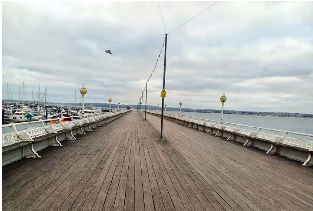
Looking down the late 19th-century Princess Pier.
