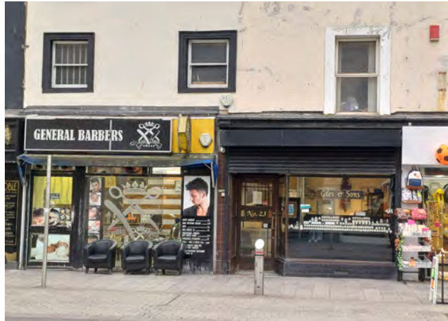
Two contrasting shopfronts on Fleet Street. The shopfront to the right retains some traditional features including a stallriser and recessed entrance door. Historic tiles denote the entrance to the shopfront from street level. The shopfront on the left has an oversized fascia, detracting window stickers and an expansive modern glass frontage.
