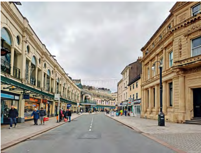
View 30: Looking north-west along Fleet Street.
