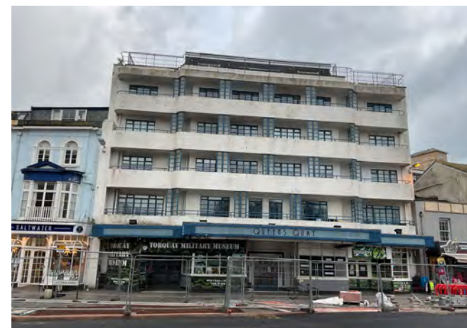
Queens Quay, since converted into apartments but originally built as hotel in the fashionable 'Art Moderne' style of the 1930s, favouring horizontal lines, rounded corners and limited ornamentation.
