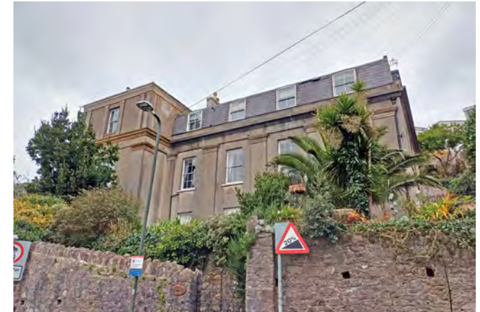
Braddons Hill House, a Georgian villa on Braddons Hill Road West.
