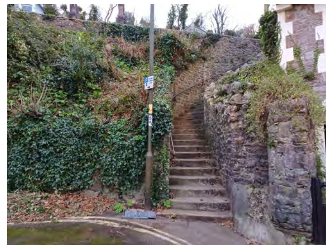
One of many important pedestrian routes within the conservation area, which lend an organic, intimate character where they survive.
