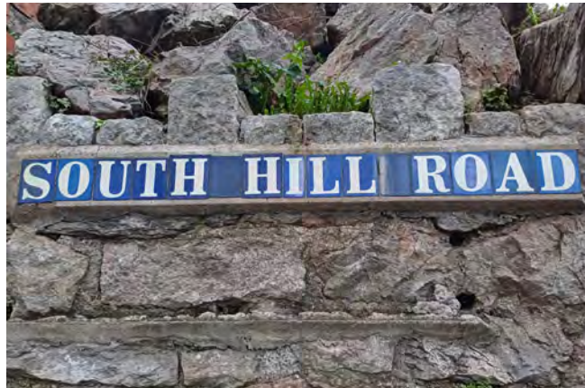
A traditionally styled nameplate. The use of small, dark blue ceramic tiles is found in many places throughout the conservation area and must once have been far more prevalent.
