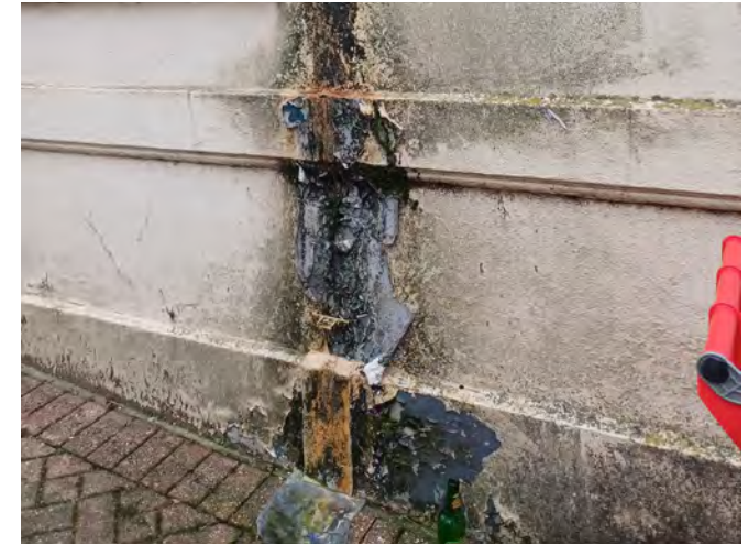
The bottom section of this downpipe is missing to a residential property on Braddons Hill Road West, which has resulted in substantial staining to the wall below.
