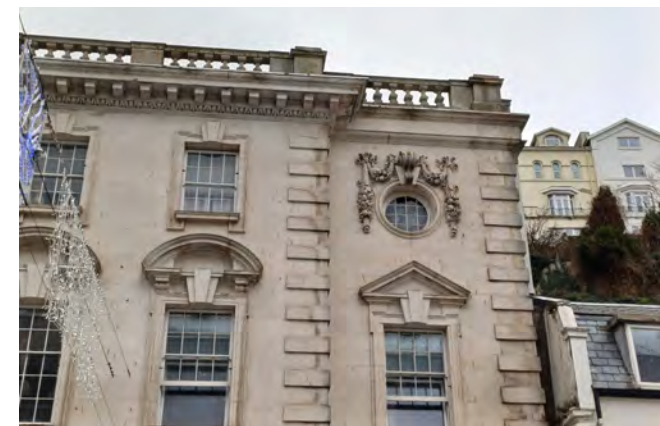
Sculptural relief articulates the primary façade of the Edwardian Post Office on Fleet Street.
