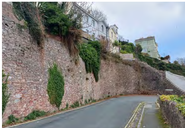
A local limestone wall along Madrepore Road.
