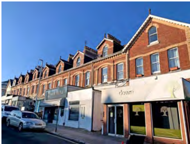
Modern 20th-century shop extensions to the front elevation to a terrace of houses on Palace Avenue. A single property in the centre of this terrace has not been extended, illustrating how the terrace would have historically appeared when they were residential houses.
