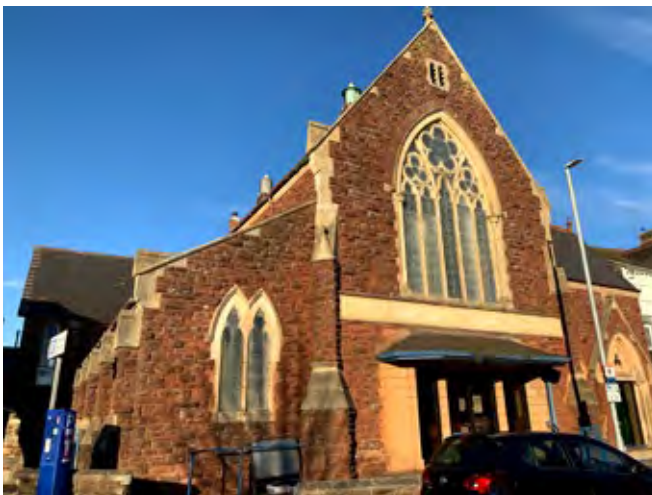
The Palace Avenue Methodist Church, constructed in local red rubble sandstone and in a Gothic Revival style.
