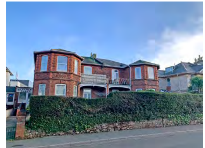
Inappropriate interventions to the balcony of a house on Dartmouth Road which depreciates the historic character of the building and the appearance of the surrounding conservation area.
