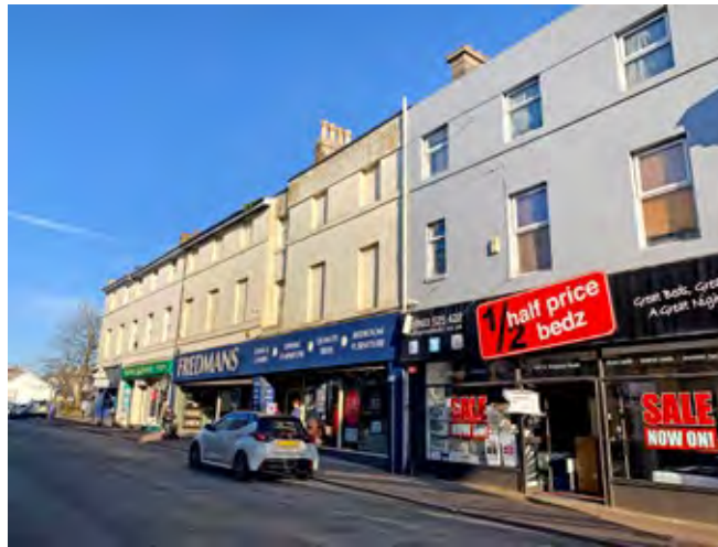
Modern shopfronts on a terrace of buildings on Torquay Road. Adaptation of these buildings for the commercial businesses has included the infill of upper floor windows.
