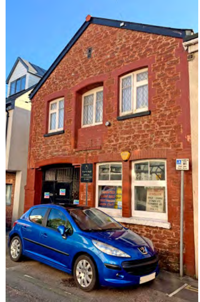
A former warehouse on Bishop's Place with ground floor rear access and a partially infilled opening to the centre of the first floor.
