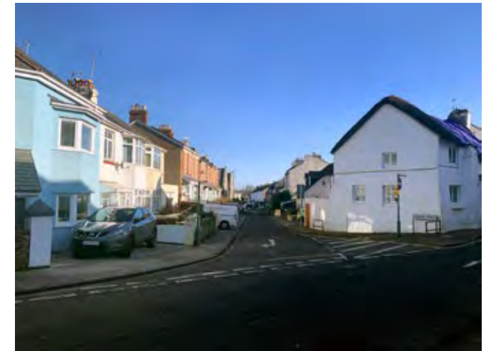
The view of Curledge Street from Fisher Street, demonstrating the variety of residential styles within the southern inner suburb of the Paignton Conservation Area.
