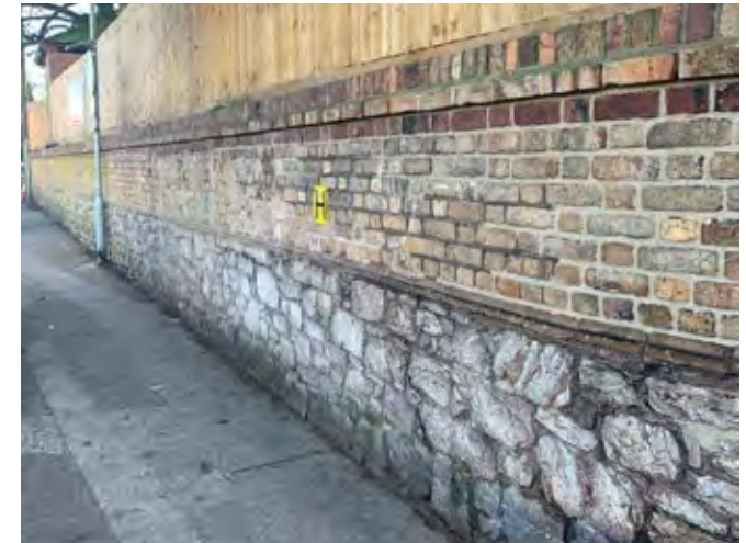
An adapted boundary wall to Tower House School on Fisher Street.
