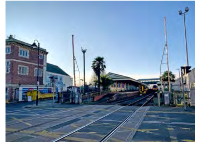
View of the station from the railway crossing, looking south.
