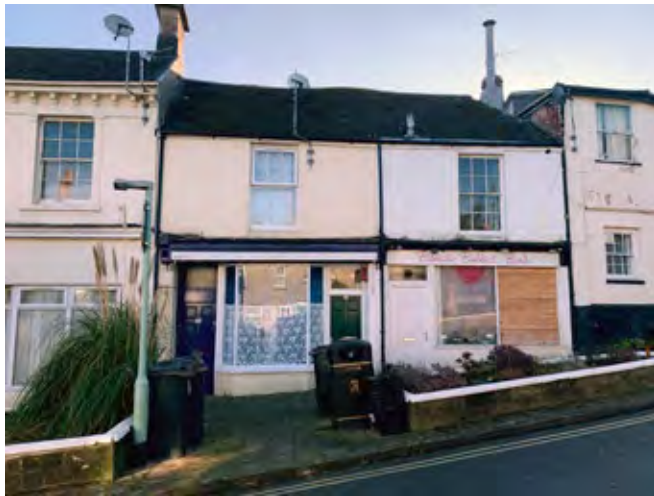
A pair of buildings on Church Street which have had their traditional shopfronts incrementally replaced with uPVC units, including the replacement of an upper floor window.
