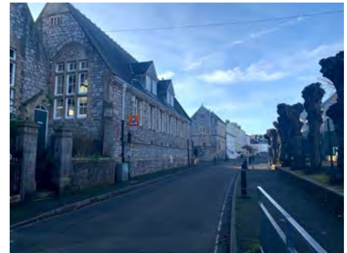
The historic Boys' School building, now a part of the Curledge Street Academy, on the south side of Curledge Street.
