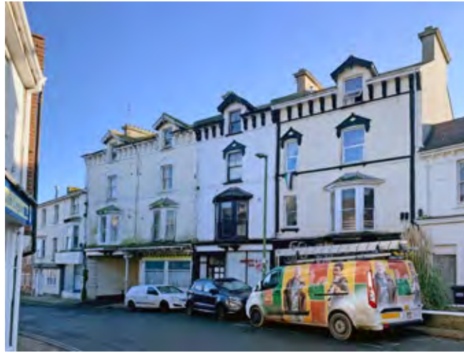
The former Crown and Anchor pub on Church Street which has been left unoccupied and been left in a poor condition.
