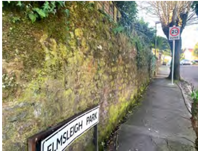
Boundary wall constructed in rubble stone to Elmsleigh Park.
