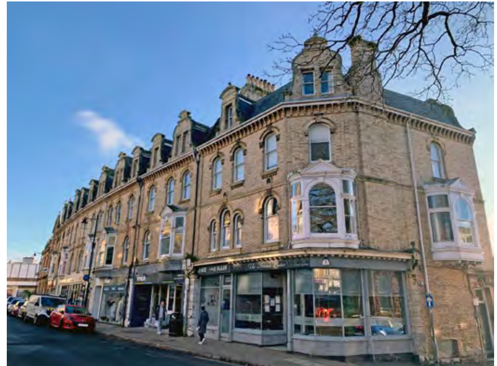
Ground floor shop units with residential housing above on Palace Avenue.
