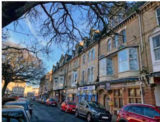
The south terrace of Palace Avenue with a range of modern shopfront adaptations and replacement windows on the first floor.
