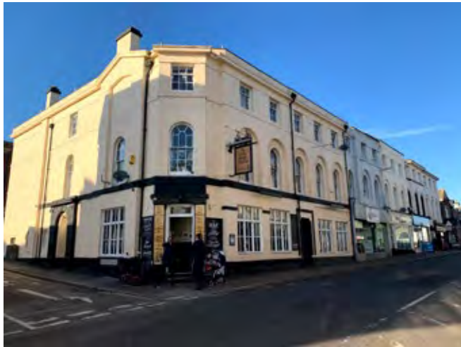
Old Well House on Torquay Road, a purpose-built inn from the 19th century.
