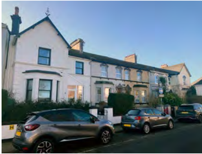
An example of a symmetrical infill terrace on Fisher Street.
