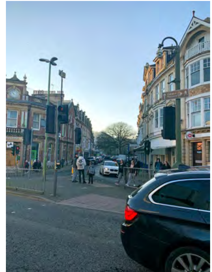
The heavily trafficked junction along Totnes Road and Torquay Road between Palace Avenue and Victoria Street.
