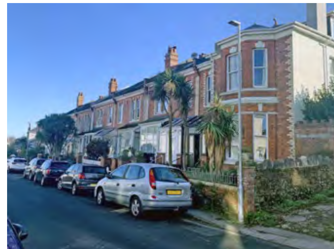
A short symmetrical terrace on Elmsleigh Road with exposed red brick, yellow brick articulation, and canted bay windows to the end houses.
