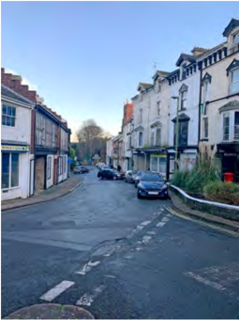
View 1: Church Street, looking east.
