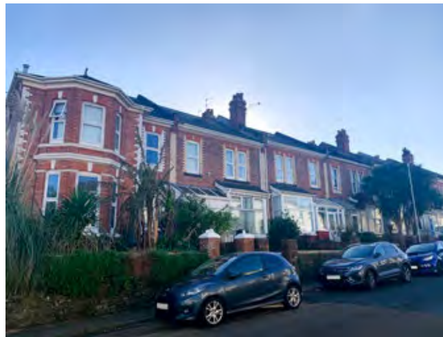
Modern uPVC sunroom extensions to the front elevation of a terrace of houses on Elmsleigh Road.
