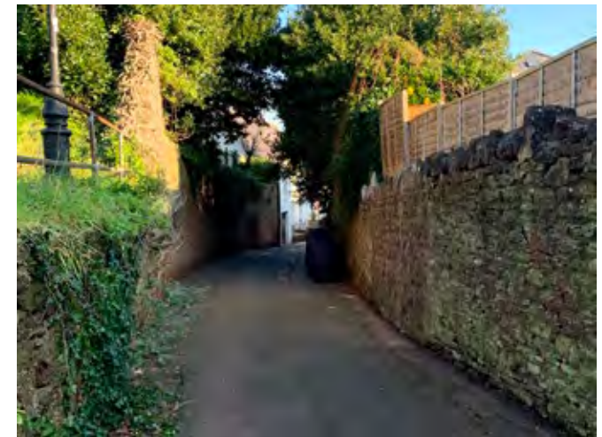
Historic red Breccia sandstone rubble boundary walls with likely medieval origins on Kirkham Street.
