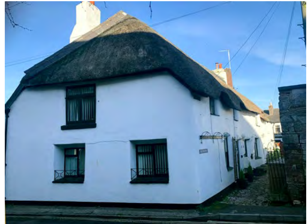
The vernacular buildings of Eaton Place, a short terrace of cob and thatch cottages.
