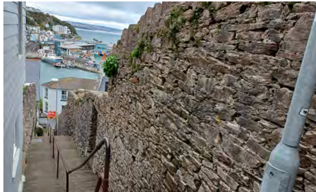
Exposed rubble stone wall at Queens Steps.
