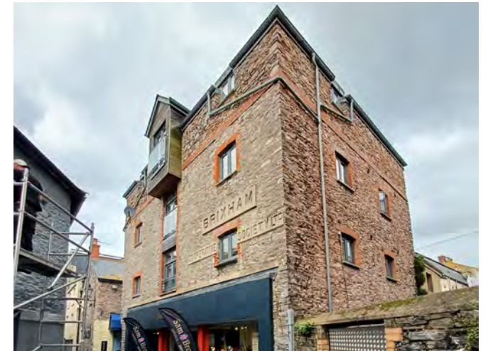
A former industrial structure off Pump Street.
