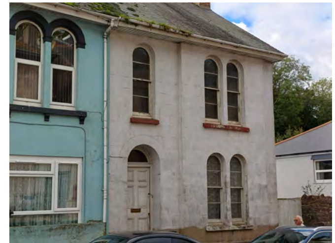
Deteriorating joinery to original windows at the end of this terrace on Bolton Street. The property is vacant.
