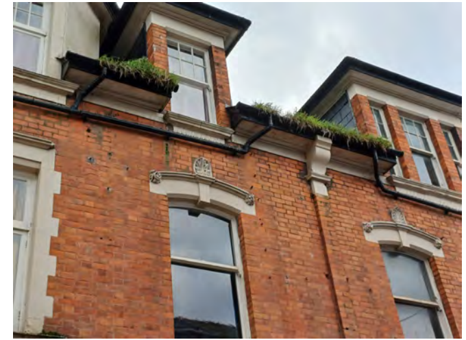
A gutter to a historic building on Fore Street, completely blocked with vegetation.
