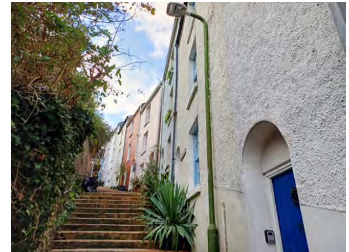
Early 19th-century terrace at Temperance Place.
