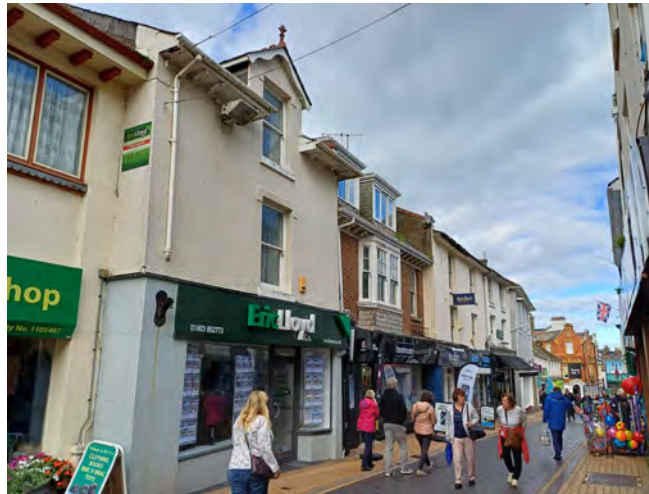
A range of historic buildings converted to provide ground floor shop fronts on Fore Street.
