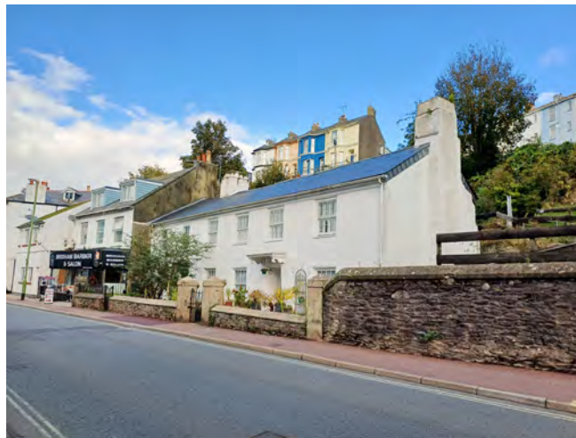
Grade II listed, early 18th-century cottages at Nos. 24-26 Bolton Road.
