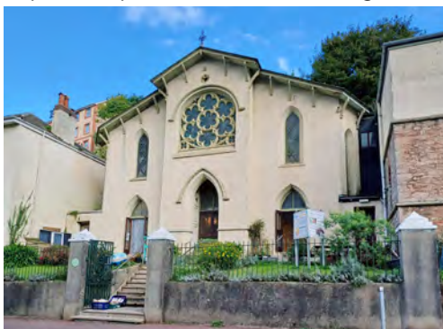
Former Independent Chapel on Bolton Street, built 1843-45.
