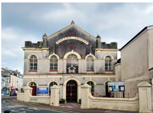
Baptist Chapel on Market Street, begun 1801.
