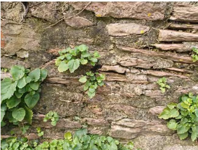
Detail of a boundary which has been repointed with non-breathable cementitious mortar and has extensive vegetation growth. A plant will typically root in mortar joints and force itself deeper as it grows, which can push the built fabric out of position and weaken the integrity of the wall.
