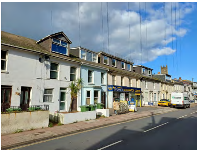
Modern box dormers disrupt the historic proportions of these properties on New Road.
