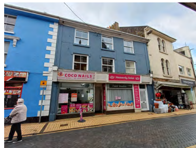
These shopfronts on Fore Street have been heavily modified through the replacement of the original window units with modern float glass and aluminium frames. Improvements might be made through the introduction of mullions and transoms and the rationalisation of advertising.
