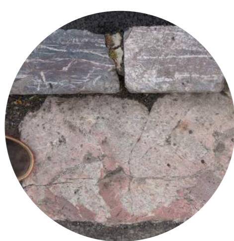
Kerbs Paving inset in carriageway to match existing
