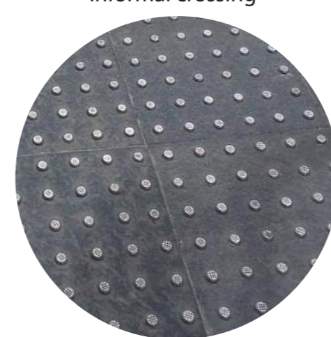
Tactiles Metal tactile studs to informal crossing points to minimise impact on public realm
