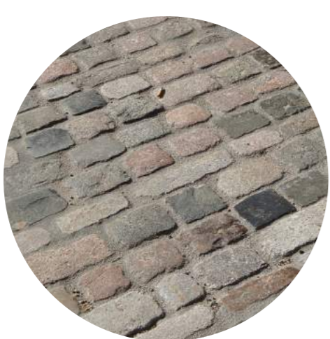
Delineation Granite Setts in Carriageway Colour Mix: violet and pinks 300mm band (100mm width units)
